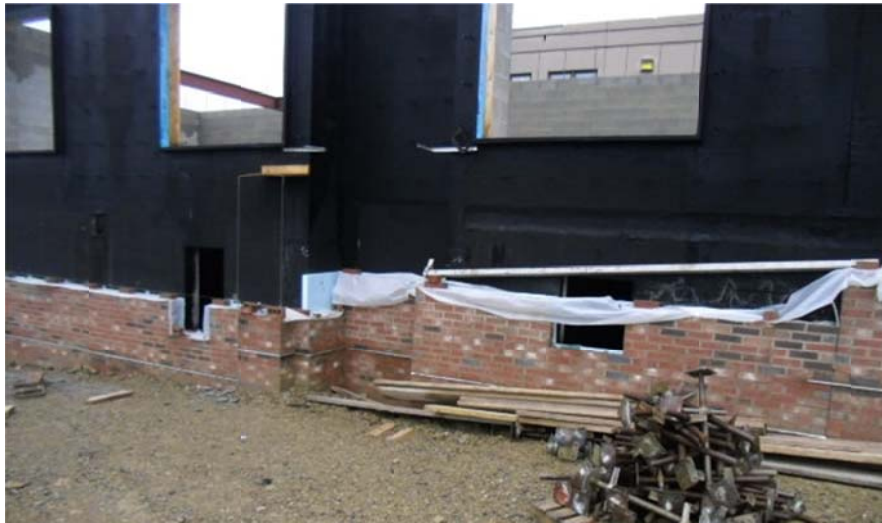
(Figure 3: Irregular Brickwork) -Courtesy of Weber Murphy Fox, Inc.
