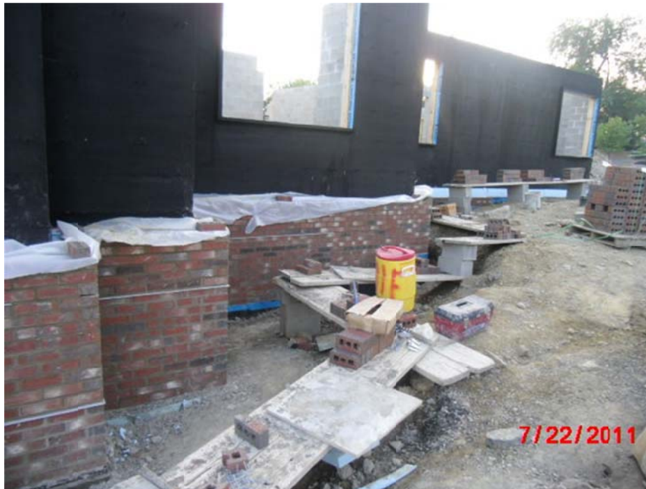
(Figure 4: Uneven Façade) -Courtesy of Weber Murphy Fox, Inc.
